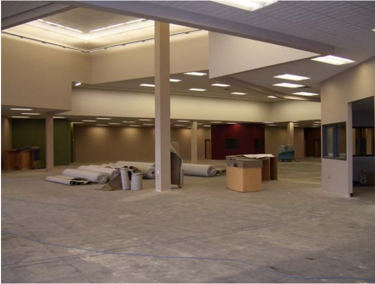
Construction of new Chugiak-Eagle River Branch Library, June 16, 2009
