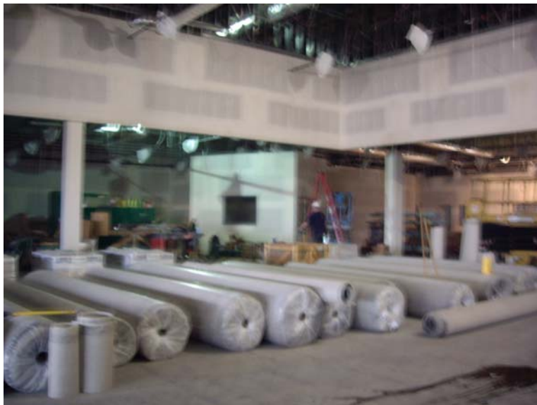
Construction of new Chugiak-Eagle River Branch Library, May 7, 2009
