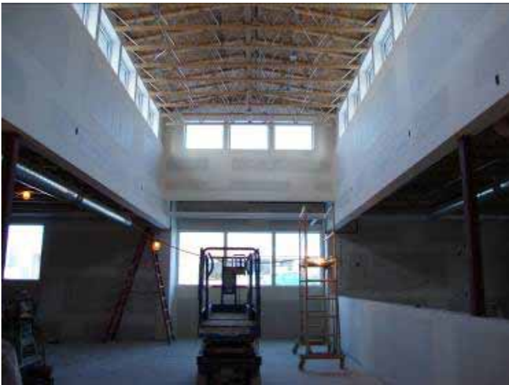
Library entrance—future site of circulation desk
