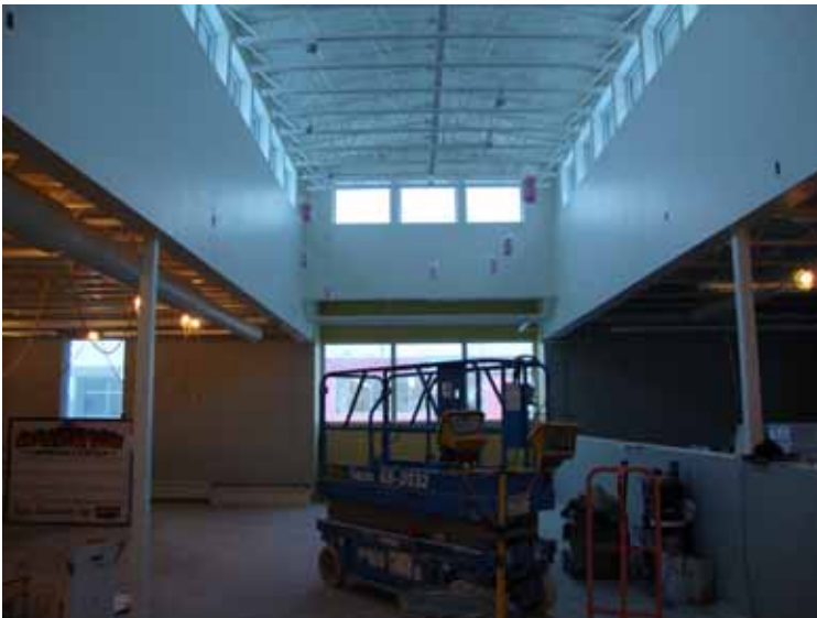
Library entrance—future site of circulation desk
