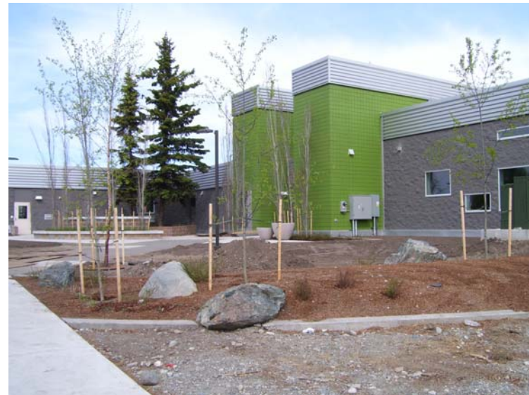
Entrance facing Clark Middle School
