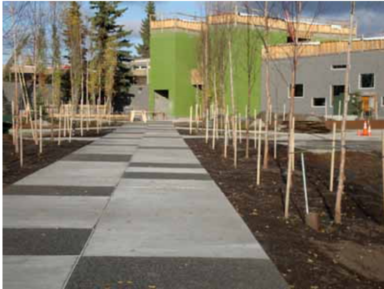
Mountain View Library Renovation, September 30, 2009
