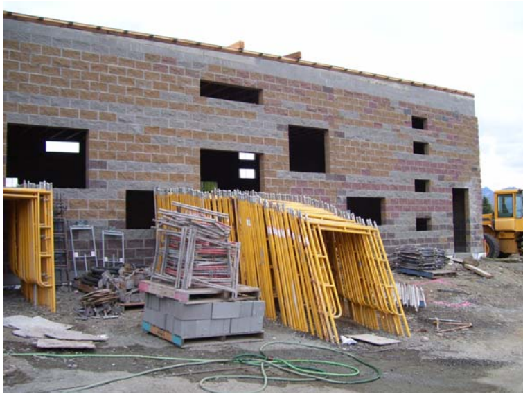
Mountain View Library Renovation, July 23, 2009
