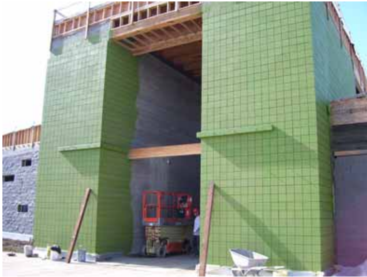
Mountain View Library Renovation, September 2, 2009
