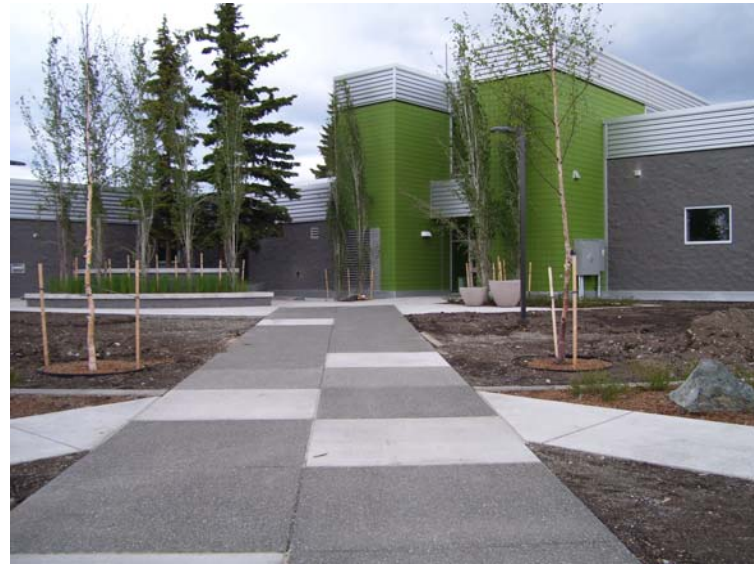
Clark Middle School side entrance
