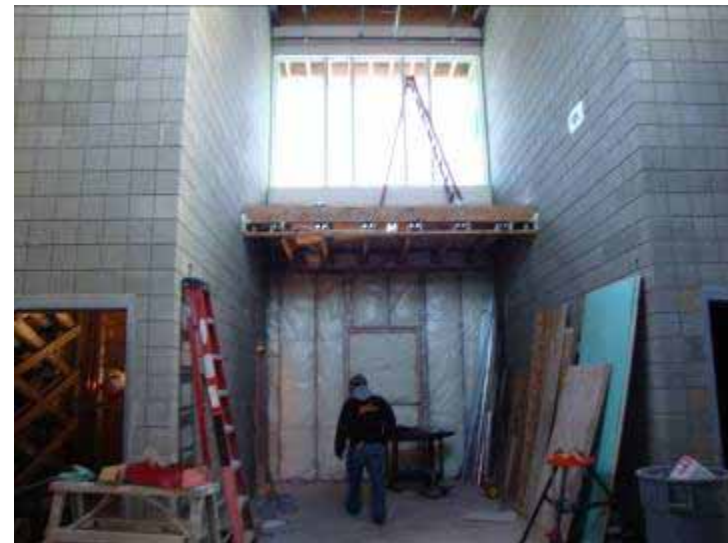
The main building entrance
