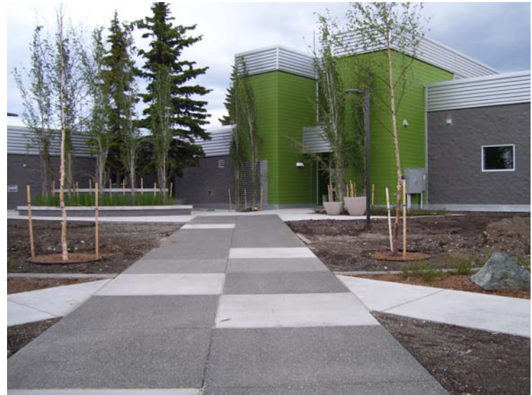
Clark Middle School side entrance
